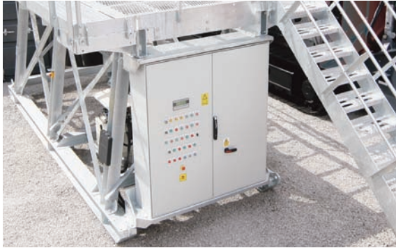
Complete Cone Starter Panel
