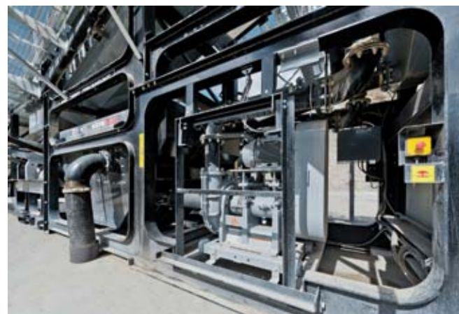
Centrifugal Pumps, Roll out for Service Access
